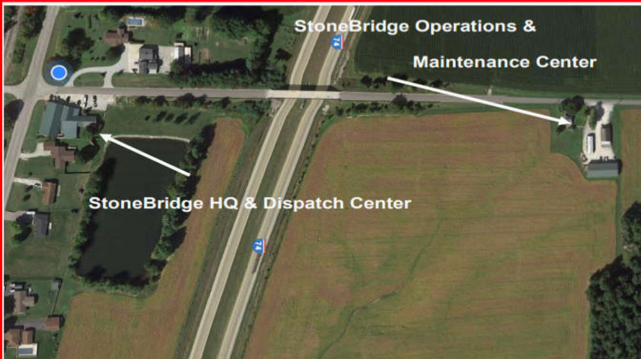
The Operations & Maintenance Center will house up to 15 StoneBridge Box Trucks
