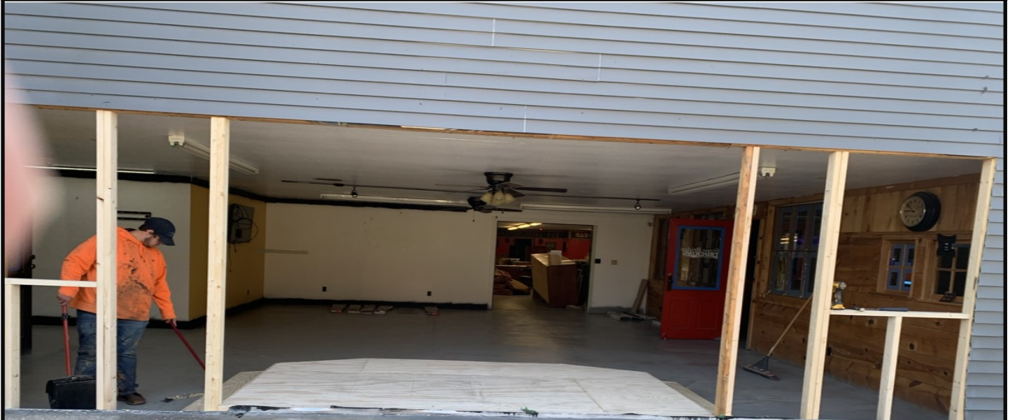
StoneBridge Operator and retired Contractor Bill Mattingly spearheaded the entire renovation. He was the lead carpenter on the entire renovation.
