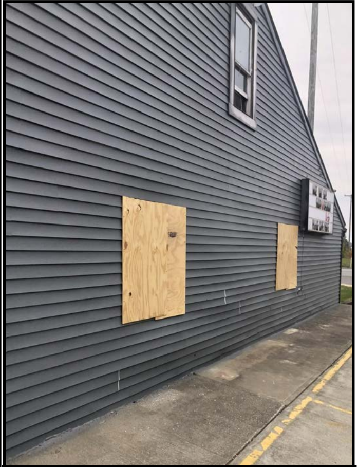
In October, the windows are boarded up in anticipation of the front door installation.
