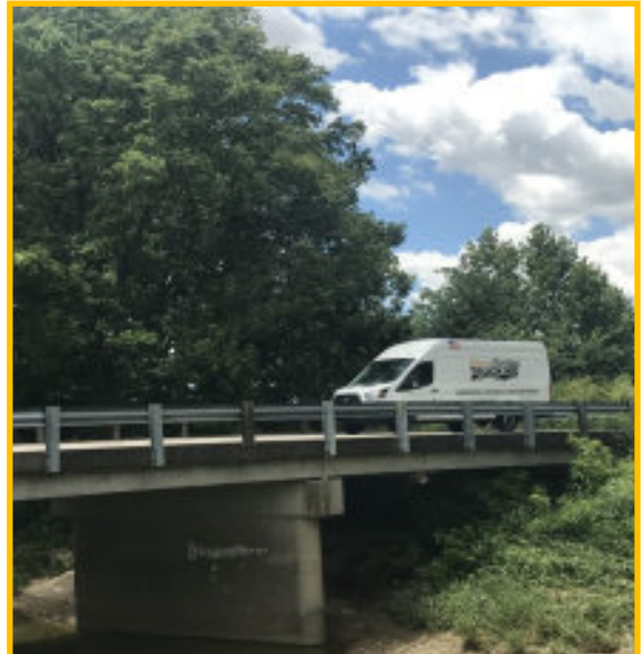
Stonebridge Transit crossing the renovated “Old Stone Bridge” outside of Greensburg, IN.
